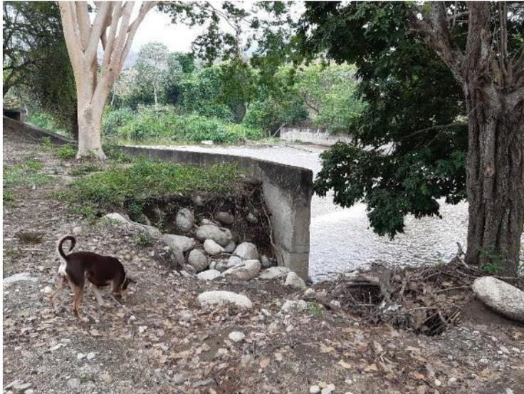
Figure 4-6 Damage to the river bank of Río Sevilla just south of the main intake of ASOSEVILLA, damage caused by the 2021 flood. (picture of Acacia Water, April 2022).
