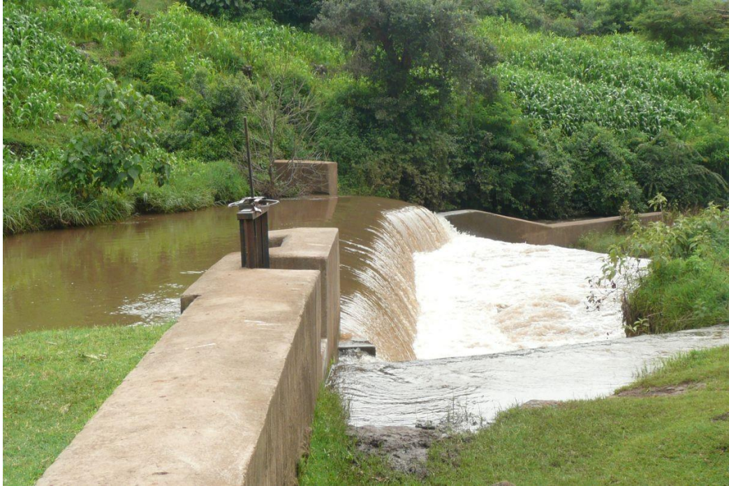
Figure 23. Typical (flood) diversion weir for water harvesting and stream diversion (photo credit: Bancy Mati, 2016)
