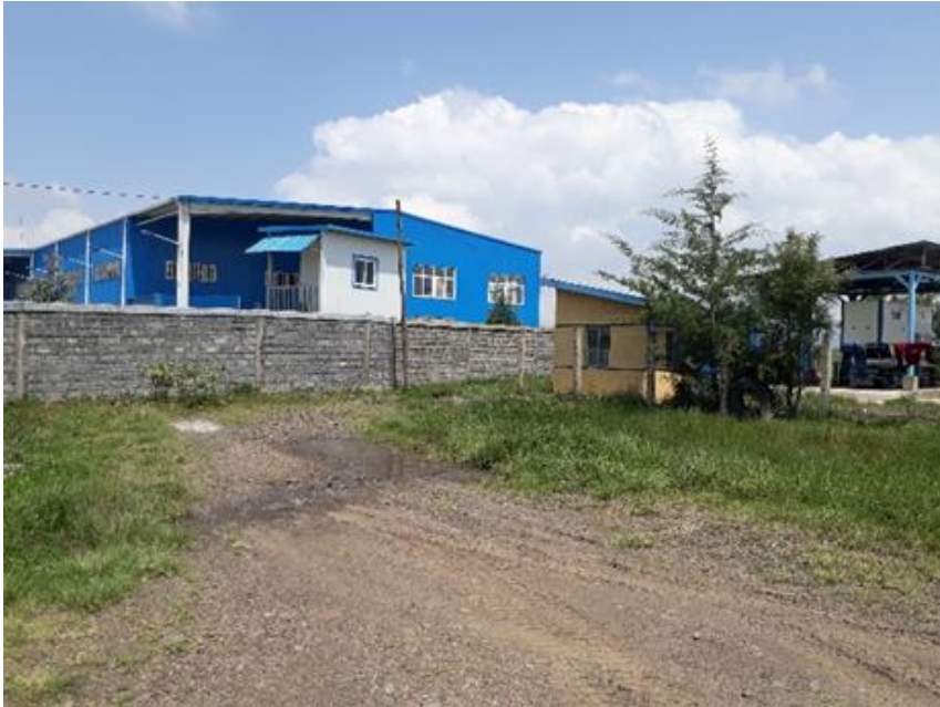
Figure 45. A mobile assembly factory very close to borehole at GPS location of 37P: 497444; 1006305
