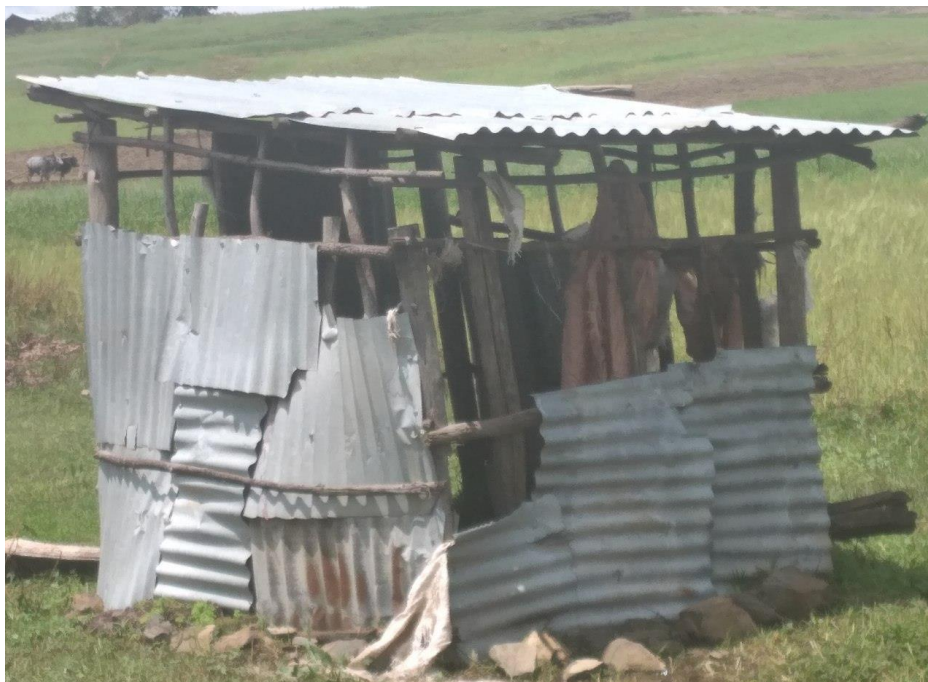
Figure 24. Public latrine in Dire rural kebele (photo credit: AquaCon, 2020)
