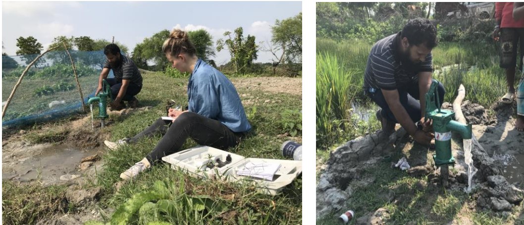
Figure 10. Photo of the flushing of exploration well RAF 1 (left) and RAF 2 (right) using a small manual handpump
