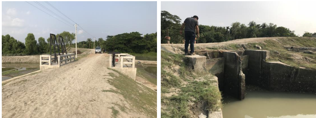
Figure 7. Photo of the new lock (left) and the old lock (right) controlling the inflow/outflow of the water in the river directly south of the site.
